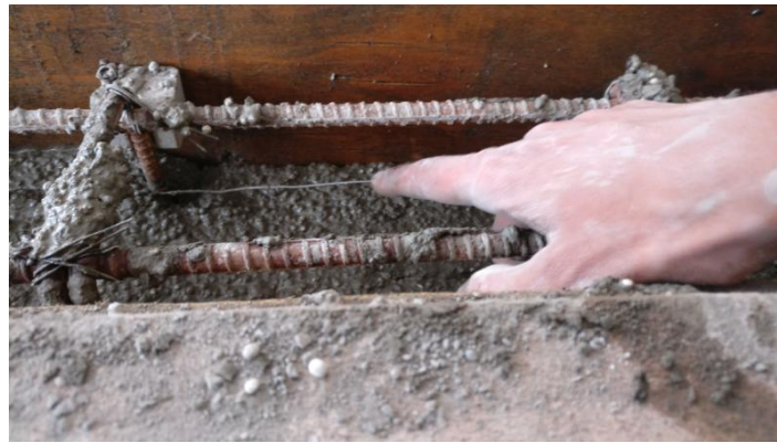
Figure 4.1 Using GI wire to differentiate concrete layers
