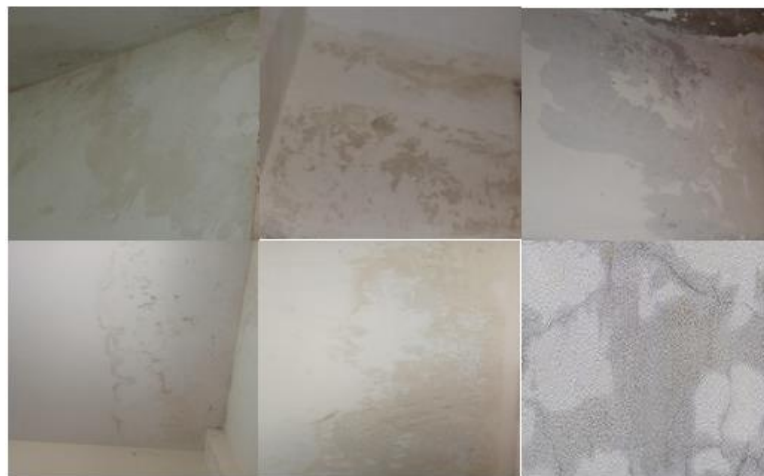
Figure 2. 3 - Seepage sample images
