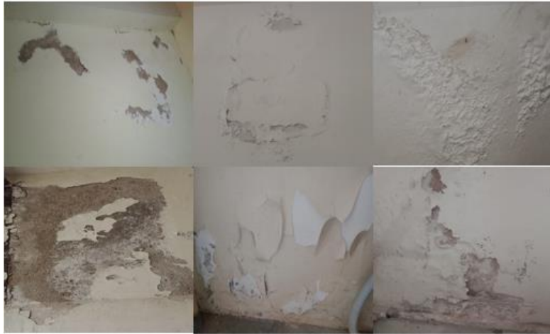
Figure 2. 4 - Dampness sample images
