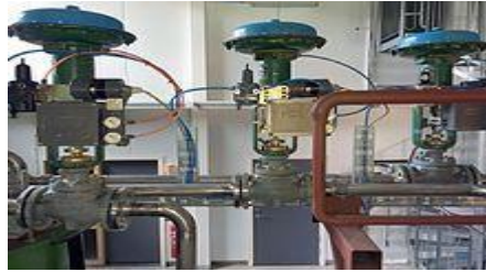
Fig 1.4 Operation of Feed Check Valve
