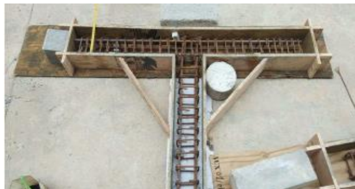
Figure Error! No text of specified style in document..4. Formwork with Reinforcement Cage
