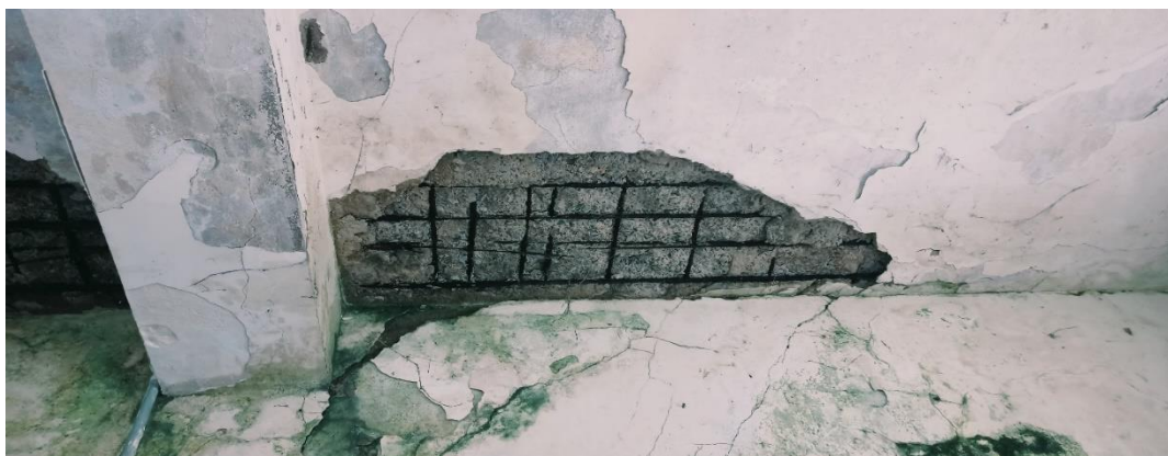
E) Cracks in Beams & Lintel
