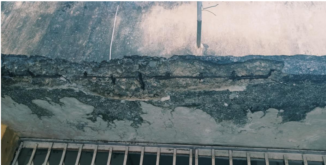
d) Cracks In Slab & Spalling of Concrete
