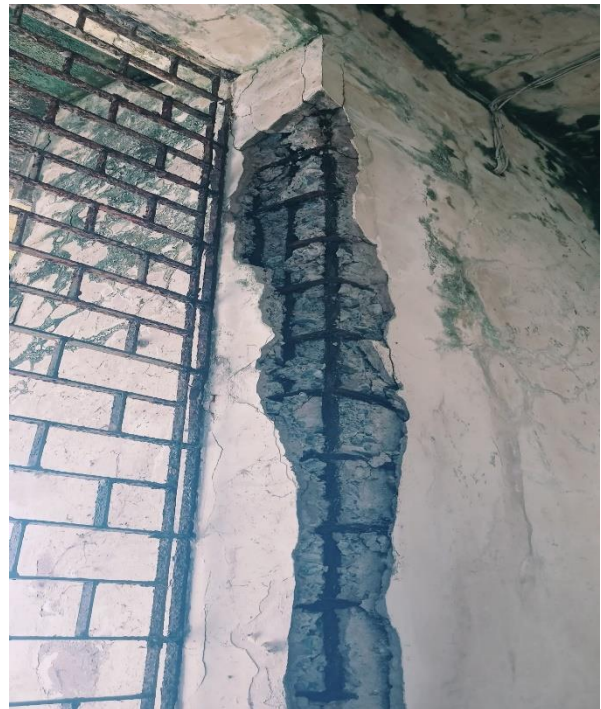
F) Cracks in Columns
