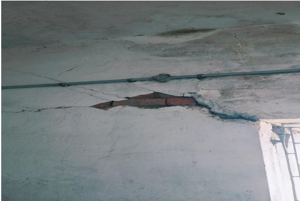
d) Cracks In Slab & Spalling of Concrete
