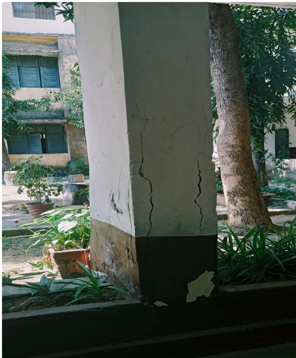
F) Cracks in Columns
