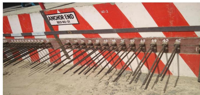
Fig. 1.4 Strands Secured at the Anchor End by Wedges
