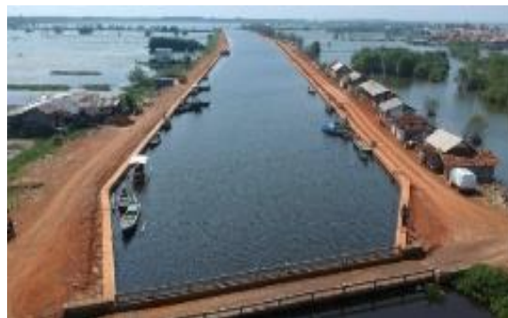
Figure 4. Protection of the Meduri River with CCSP for flood control.
