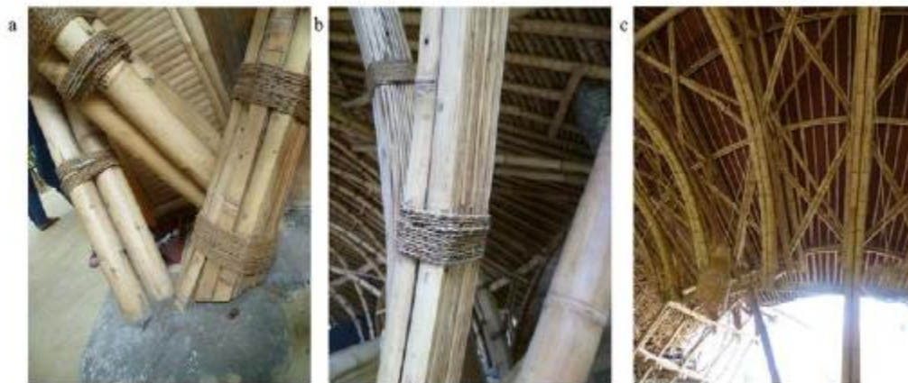
Figure 6. Bamboo connection using Tali
