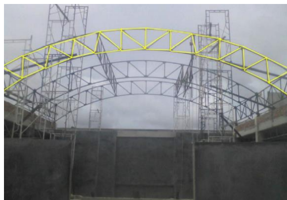
Figure 2. Truss on the roof structure
