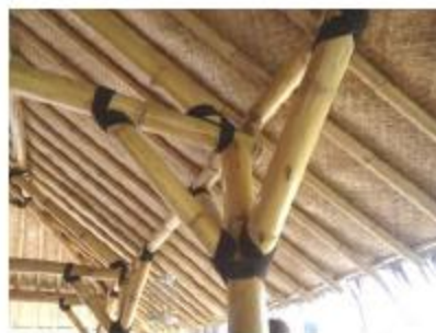
Figure 7. Bamboo connection using Tali
