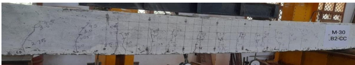
(b) Crack Pattern of B2-CC Beam
