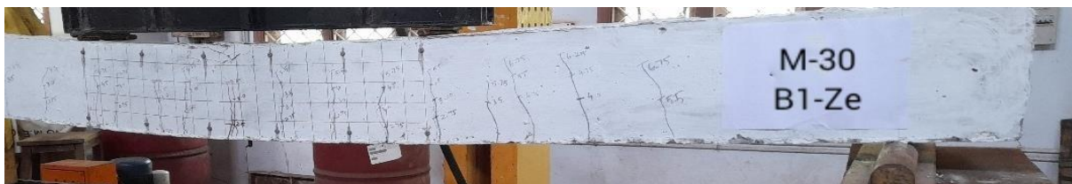
(c) Crack Pattern of B1-Ze Beam
