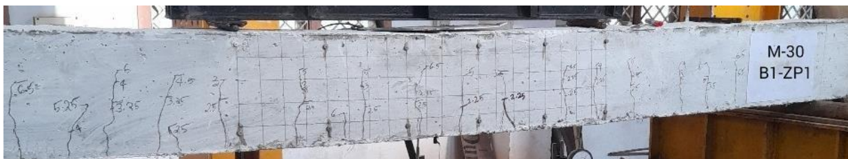
(e) Crack Pattern of B1-ZP1 Beam
