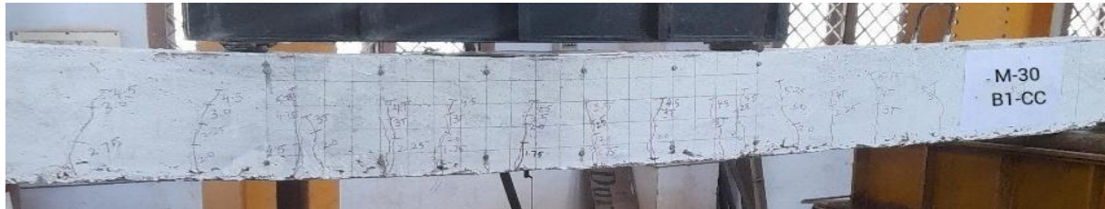
(a) Crack Pattern of B1-CC Beam
