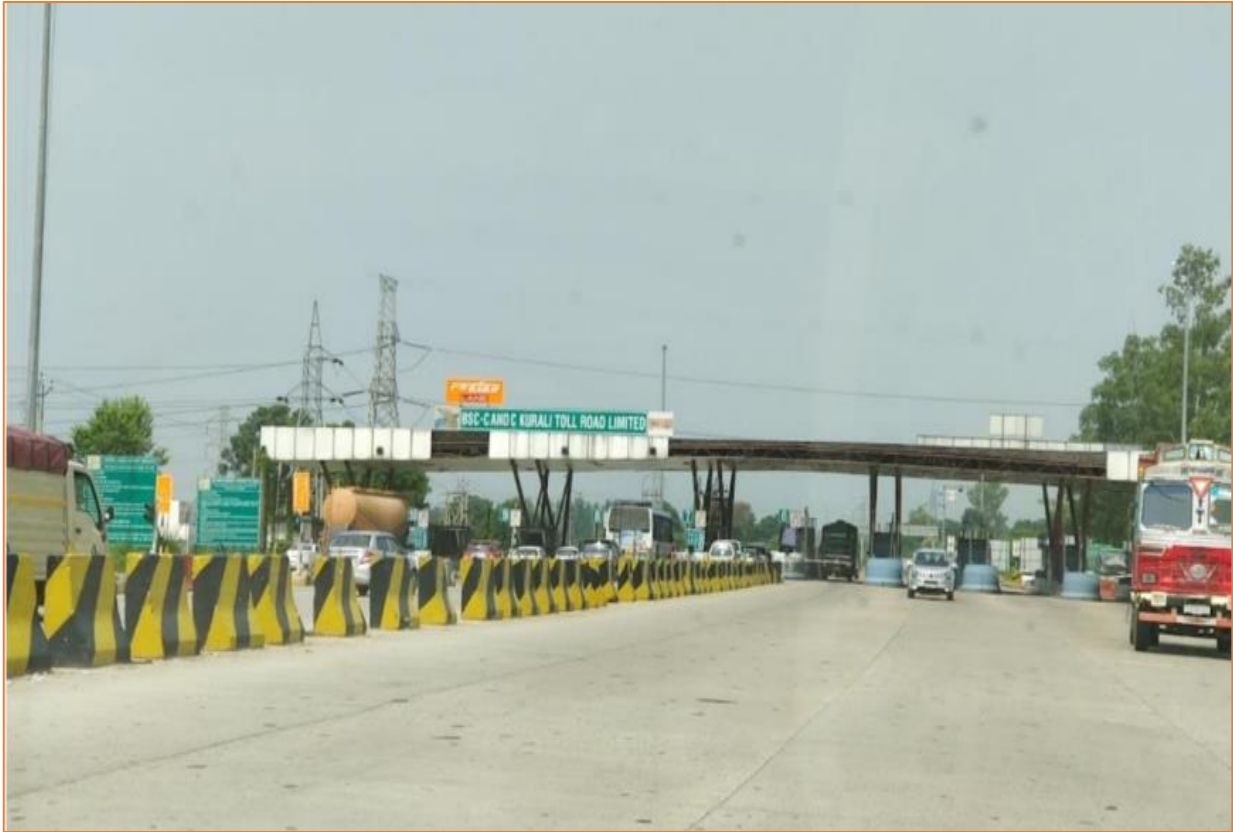
Fig. 3: Behrampur Toll Plaza On NH-205 (10 Lanes).
