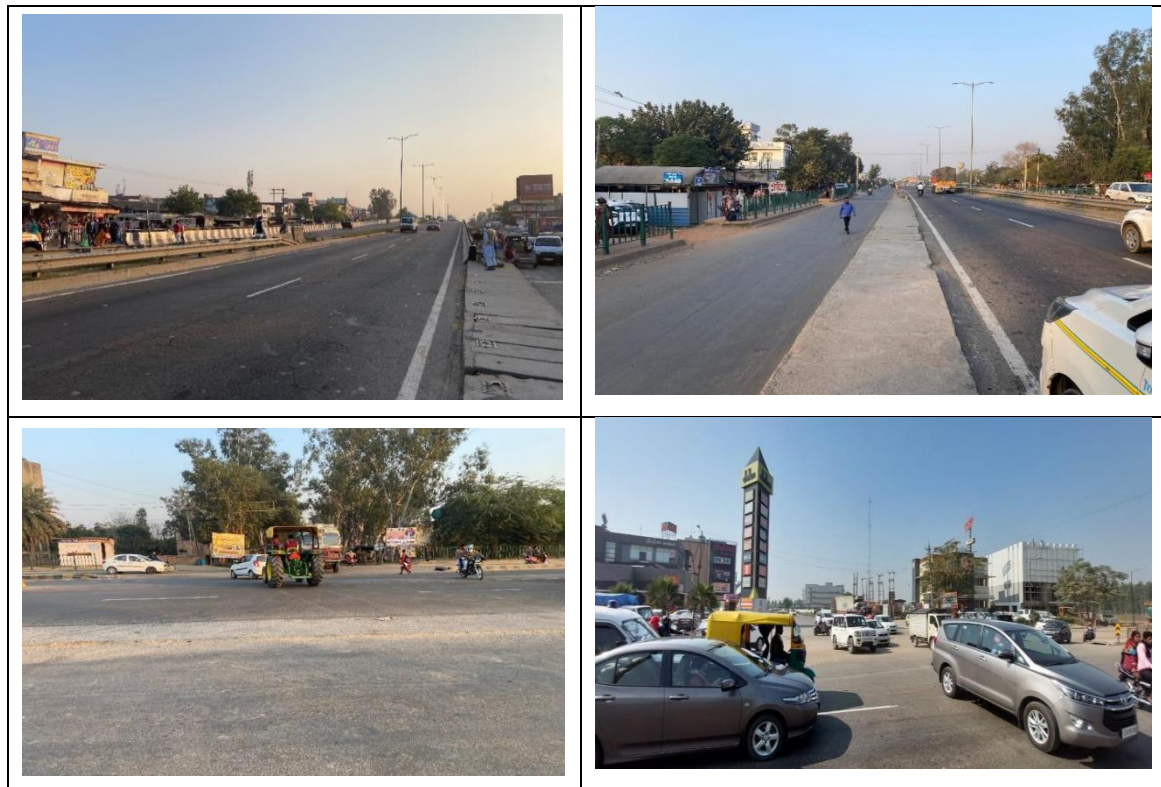
Fig. 7: Black Spot Location due To Entry and Exit Point At Near SBI Lalru.
