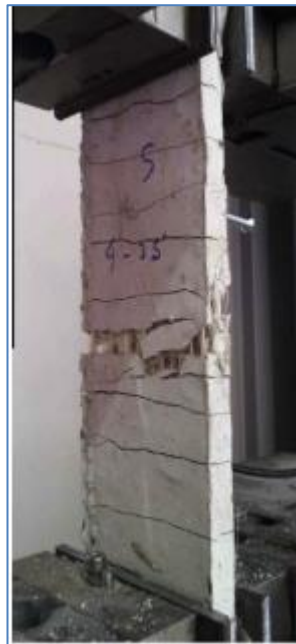
Fig. 11 Tensile test specimen failed after TRM [26]
