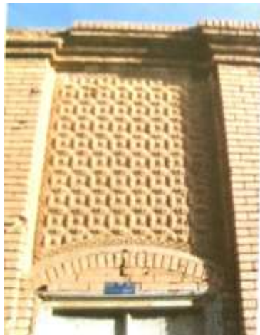
Image 32: Kolah Farangi Neighborhood portals (Bricklaying design and use of Mohri bricks on the cymatium; stretcher bond in the arched stringcourse framing in the lintel) (Source: author, 2020).
