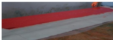
Fig 6: Applying of matrix
